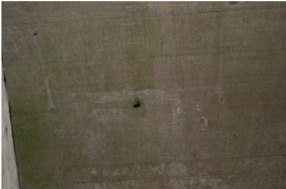
Plate 4 – Bridge 2 – Bridge carrying M1 showing drainage pipe in wall of bridge
