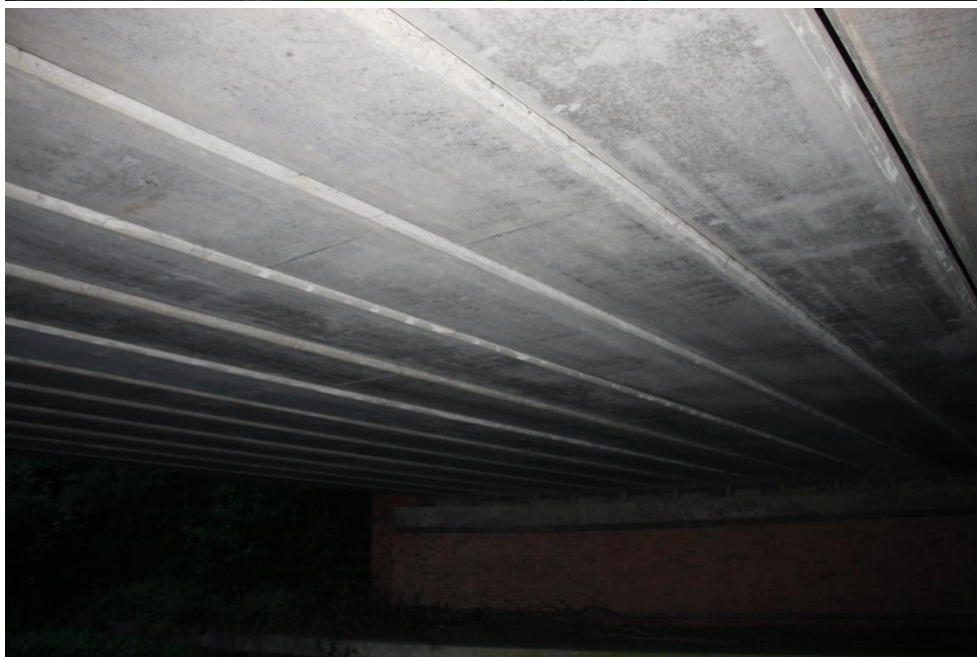
Plate 6 – Bridge 3 – Underside of bridge showing gaps between deck sections.
